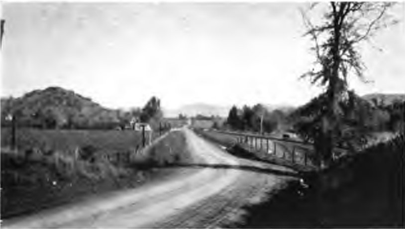
A rerouting of this State Highway line eliminated two grade crossings. Old road to right.
